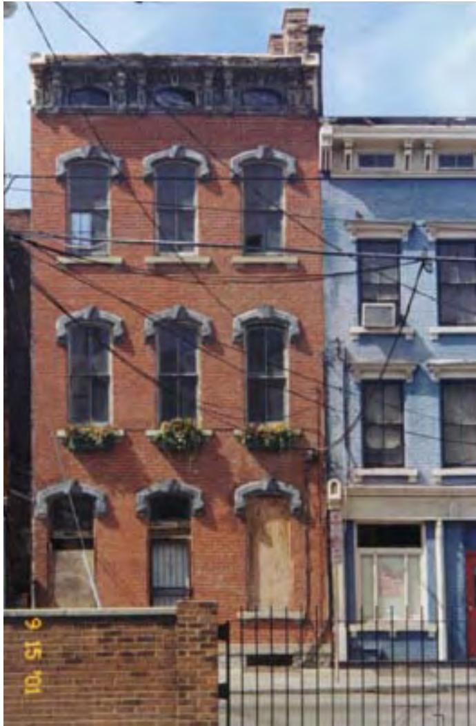
Figure 24: Housing in the process of rehabilitation. Photo courtesy of Julie Fay.
