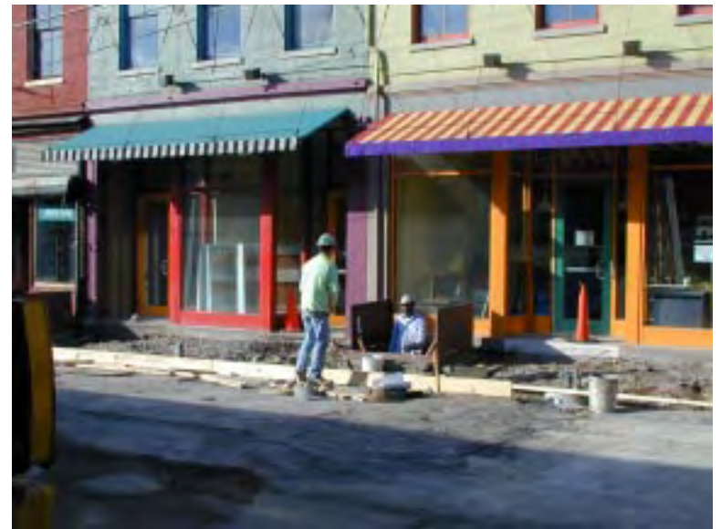
Figure 77: Improvements being made to the buildings surrounding the Market House.
